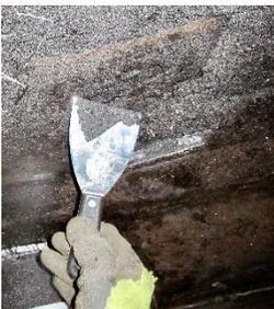
1. The repairs must be only in one spot (like our vent,) and not spread throughout the tank.
